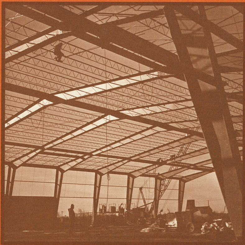
Above: Steel work is erected for the new Physical Education and Recreation Center on the Eisenhower campus.
